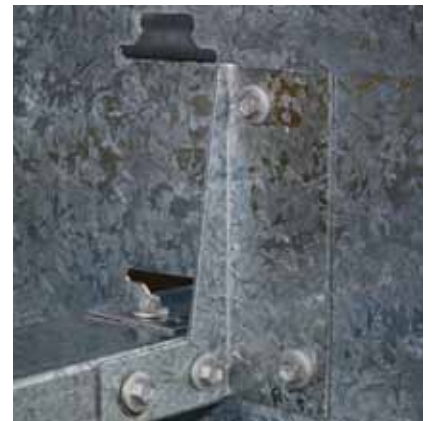
BRIDGE BAR STABILISER Prevents purlin roll
