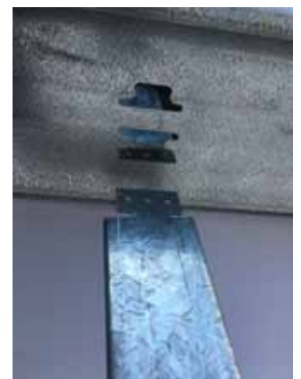
PURLIN KEYWAY Simple roofing screw assembly
